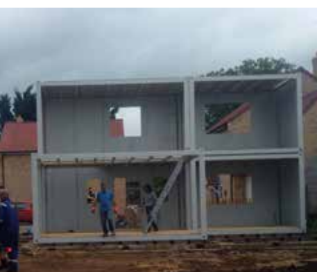
Crane placement of modules
