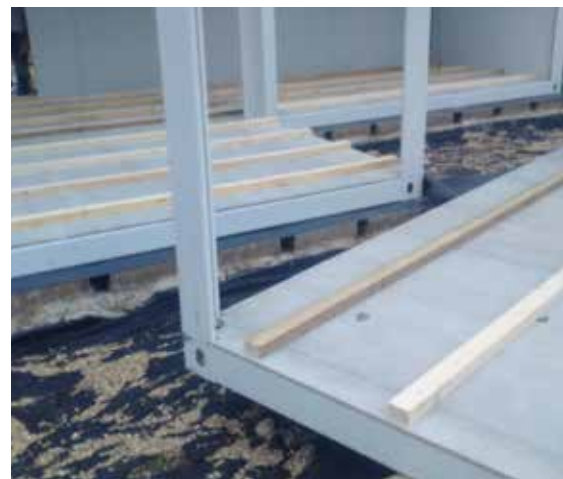
Module placement on 10kN blocks
