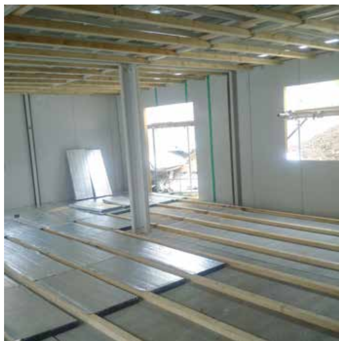
Insulation under floating floor
